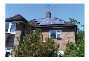
This 1.44 kWp solar photovoltaic (PV) system was installed in Cambridge in June 2010. It is a relatively small system making good use of an awkward area of roof. The use of space was optimised by installing panels 'landscape' as opposed to the more usual 'portrait' positions as well as stepping the array with the shape of the roof.
